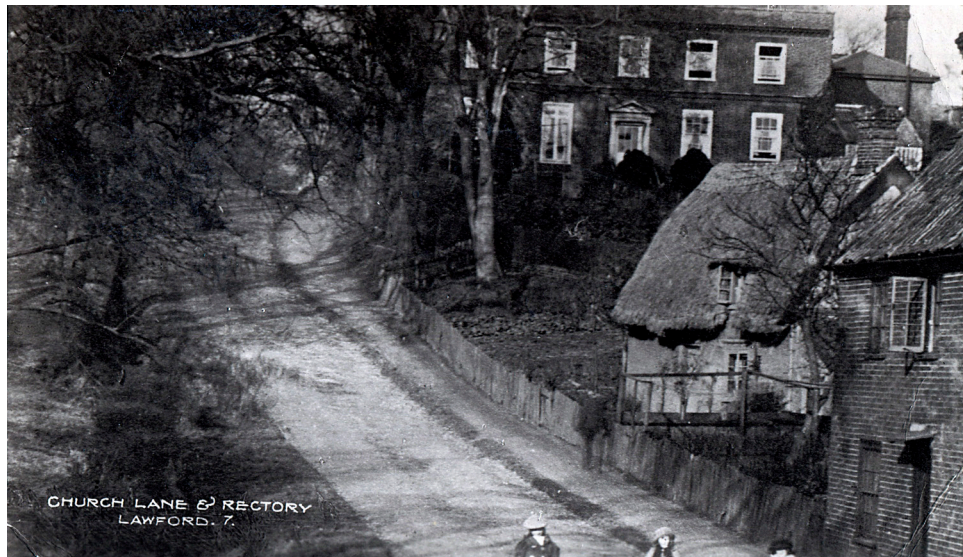
Figure 5 Photo of Church Lane, Rectory
